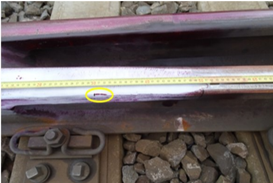
Longitudinal cracks on other running surfaces of the casting Defect code 622N
