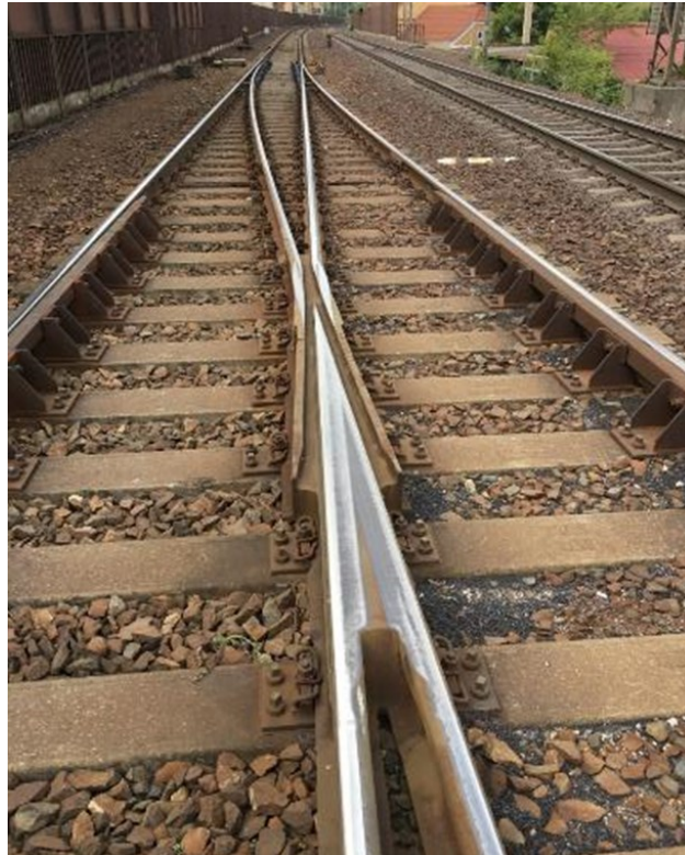
Figure2 - Frog in the switch in the track
